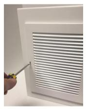
Take off wrapper from Register Insert. Place the Flap Damper Register Insert into the Baseboard Frame, with the damper control on top.
